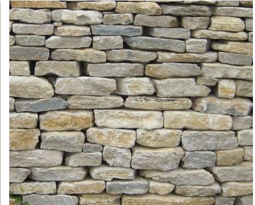
Rubble Stone Wall Image courtesy of https://www.anbentonweatherstone.co.uk/products/purbeck-rdom-walling-on-flat
