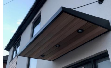
Canopy with aluminium fascia and timber soffit
